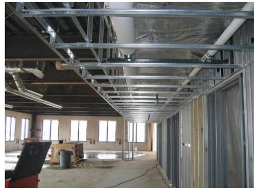
The revolutionary ShortSpan tee's "peak-form bulb" adds strength, allowing you to eliminate more than half of the supports to structure required using traditional framing methods and materials.
