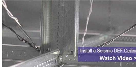
Armstrong's Seismic Wall Angle provides an additional 1/4" of bearing for tees while preserving the 3/4" float clearance required by code between the end of the tee and the wall. Seismic RX allows the elimination of 2" wall angle and stabilizer bars, as long as Armstrong's Beam End Retaining Clips (BERC2) are used. The BERC2 clips hold tees in position, while allowing for lateral motion. The BERC2 clips can also be used on the fixed wall tee ends to eliminate pop rivets.
