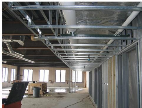
ShortSpan will support spans up of to 8'-6" with no independent support, and spans of up to 17' with StrongBack or Locking Pocket Main down the middle of the span. The system is engineered to save time on installation, with these features:
